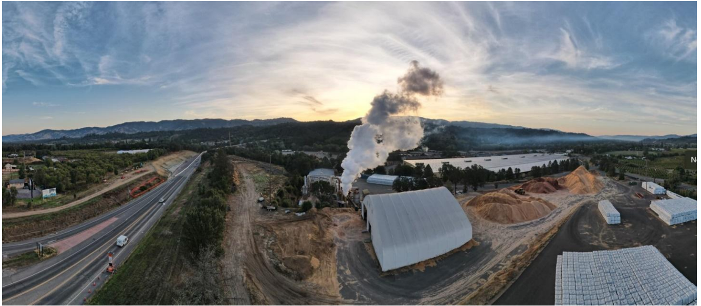
Calpella pellet plant, credit Juan Mejia
